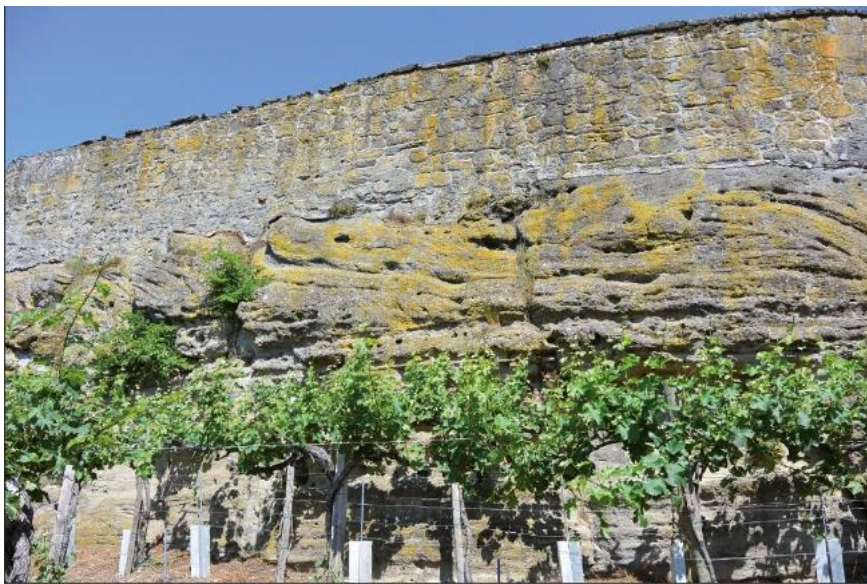
Fig. 28: Slip folds in the base sediments at the beginning of the maar lake stage in Riegersburg
